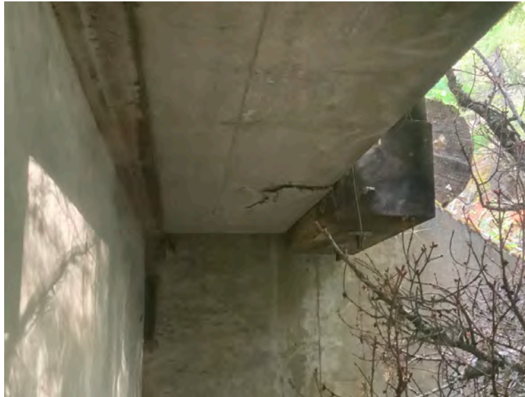
Deck, first panel right bank
