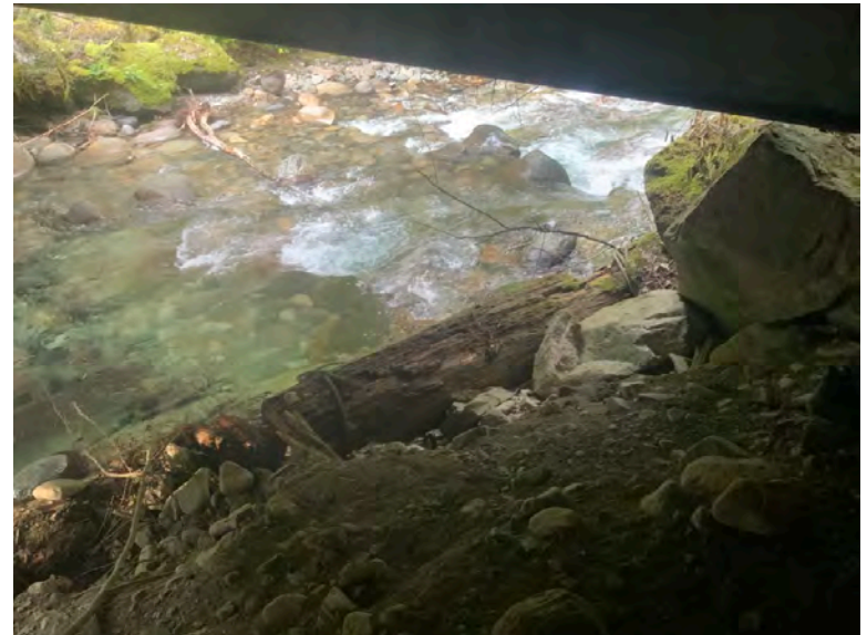
Right Bank Abutment when facing downstream
