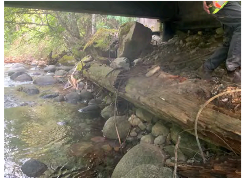
Right Bank Abutment when facing downstream
