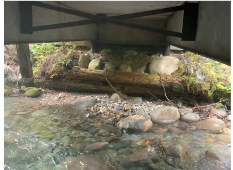
Left Bank Abutment when facing downstream
