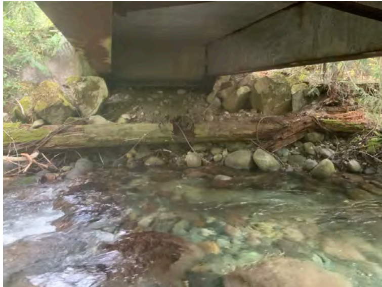
Right Bank Abutment when facing downstream
