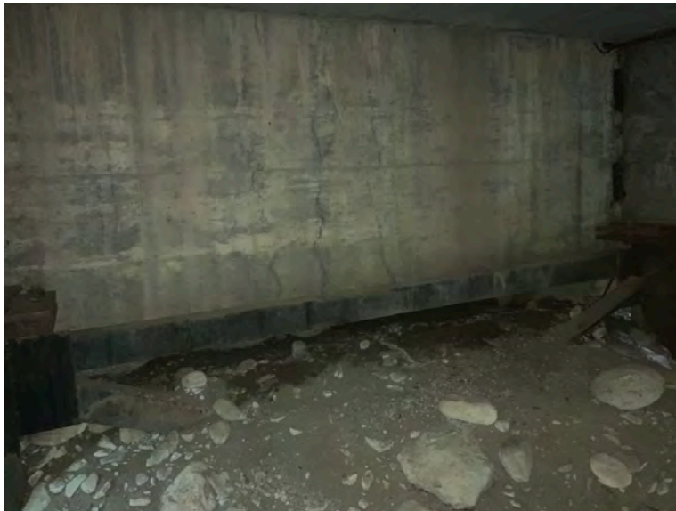
Right Bank Abutment when facing downstream
