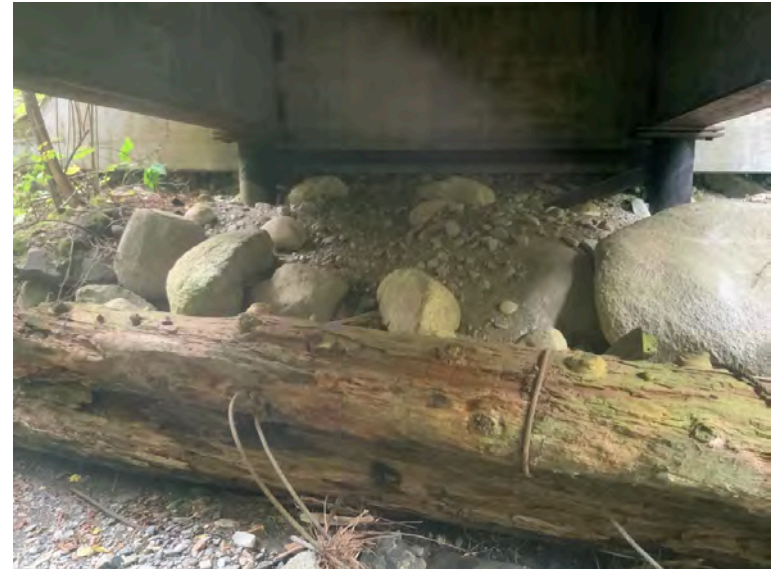
Left Bank Abutment when facing downstream
